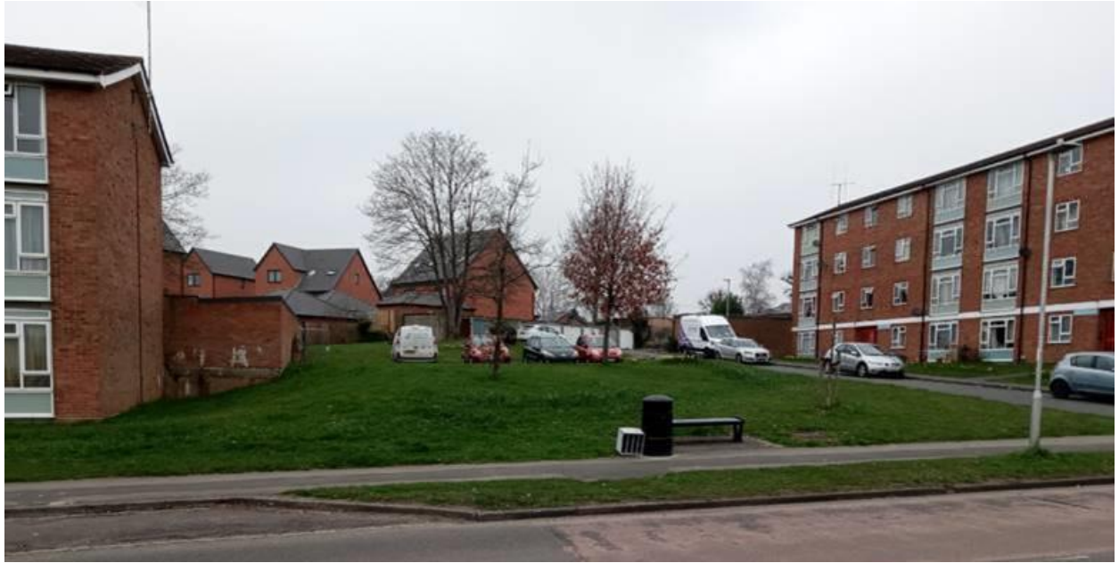
Site photograph from Wensley Road
