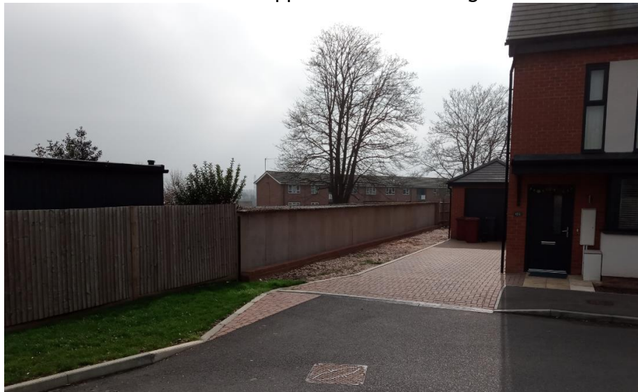
Existing rear elevation of garages from Coley Avenue
