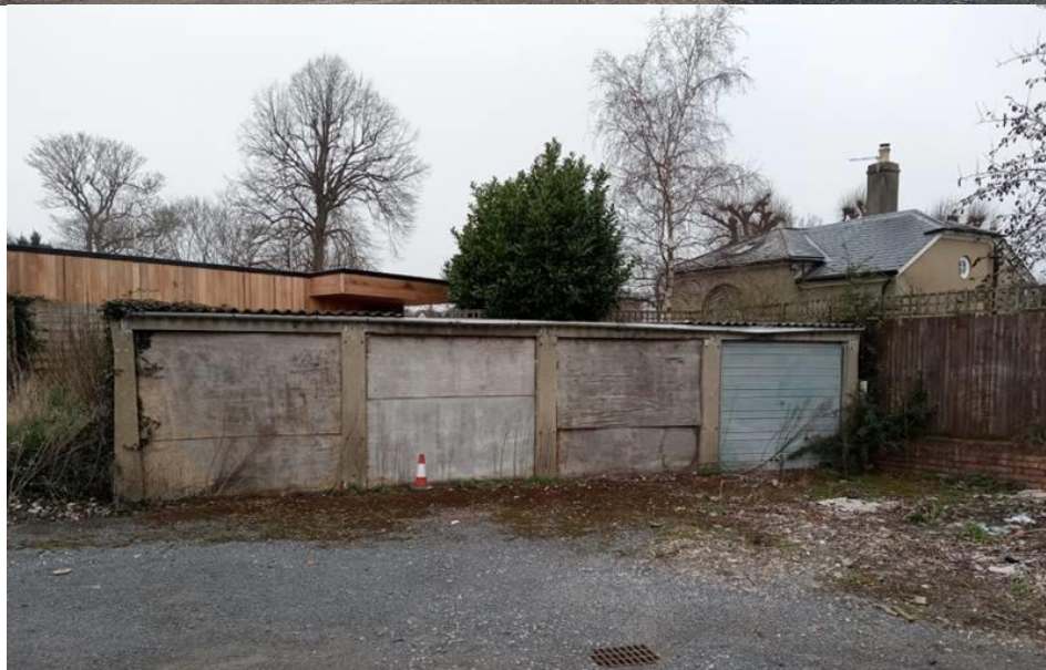
Existing garages (East Lodge listed building in background)
